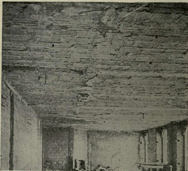
FIG. 40. — Interior of Chesapeake & Potomac Telephone Building, Baltimore Fire.
